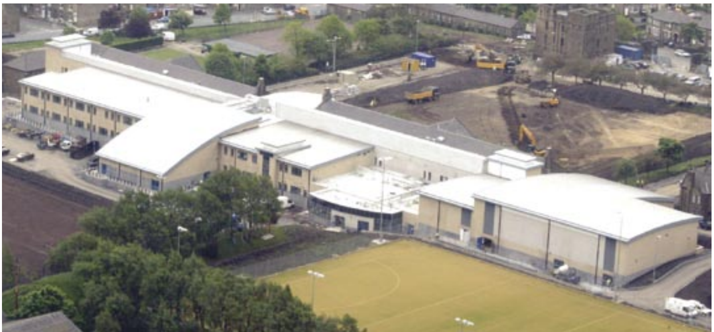
Works almost complete at Halifax High School, part of a £3 million contract for Calderdale PFI Schools.
