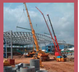
Above: The lift of the main 44 tonne trusses in progress.
